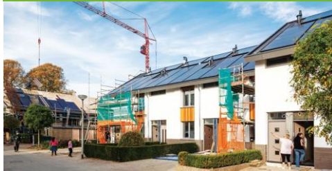
Intelligent district renovation
